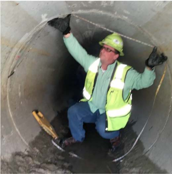
FIG. 1 Person Entry Inspection
