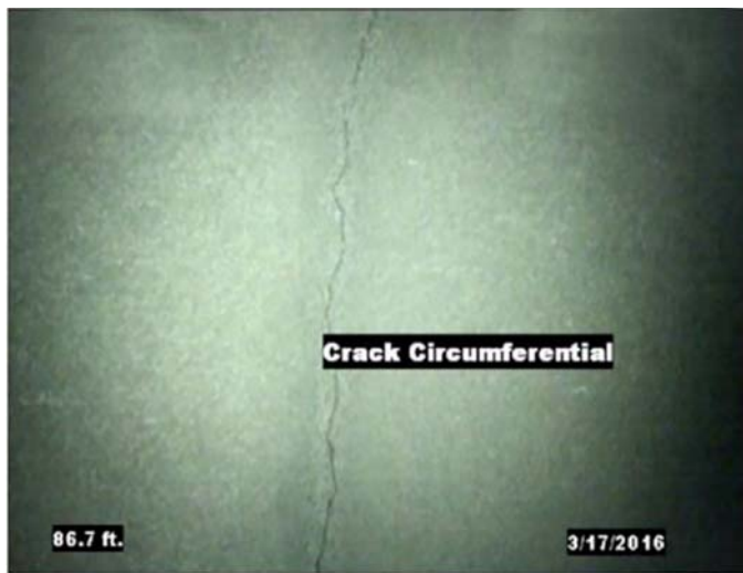
FIG. 6 Circumferential Crack
